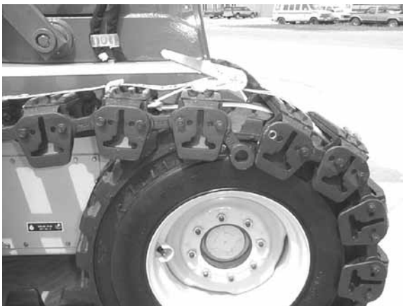
9: The skid steer will have to be driven back and forth to ensure a majority of the slack is taken out. Be careful not to drive too far, as damage to web binder or skid steer might occur.
